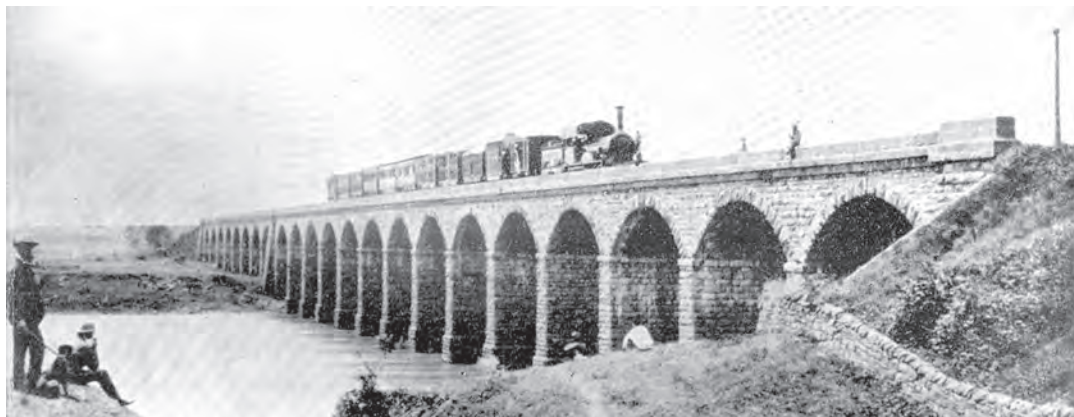
Fig. 1.4 First Railway Bridge linking Bombay with Thane, 1854
