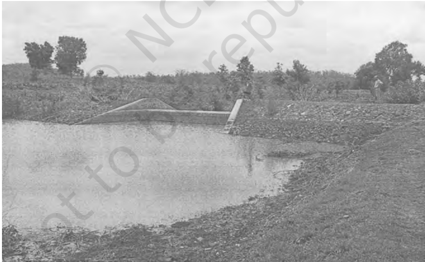
A small dam
