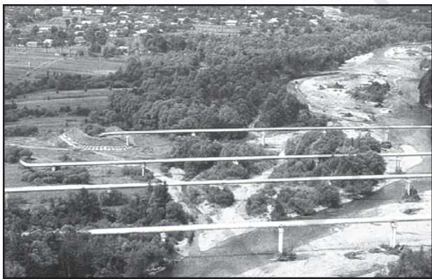
Fig. 7.17: Pipelines transporting natural gas in Ukraine
