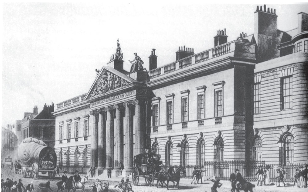
Fig. 17 – East India Company House, London.
